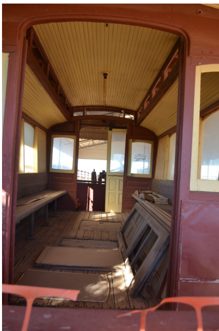
Before work started on the Tram in June 2014.
