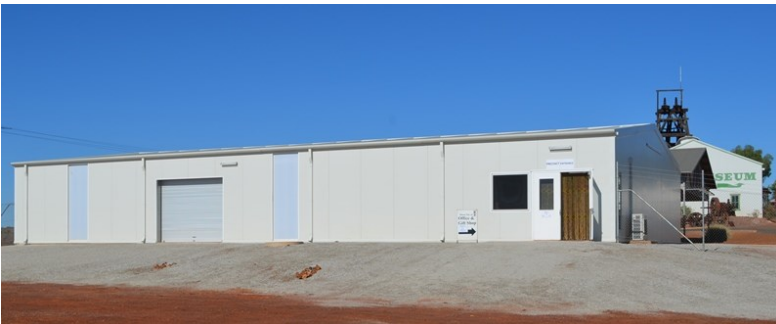
The western wall of the new vintage vehicle shed.
